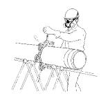
Blade cutters are frame adjustable to the circumference of the pipe and have a number of self-tracking rollers that align one or more carbide-tipped cutting blades. Because of the relatively low mechanical input and clean cutting action, hand operated blade cutters do not produce significant amounts of airborne asbestos dust.
